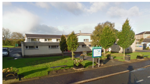
Fig 2: The Site in 2009 with the previous structure
